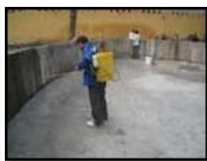
Water Park of America, Bloomington, Minnesota: Crystal Lok® applied onto concrete tanks during winter maintenance.
