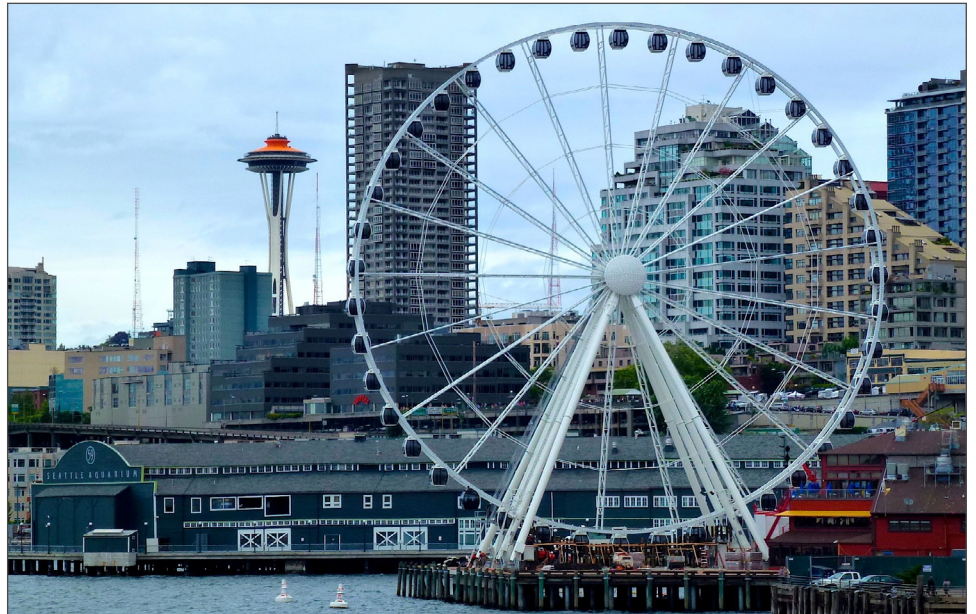
Helix Micro-Rebar replaced rebar cages in Pier 57.
