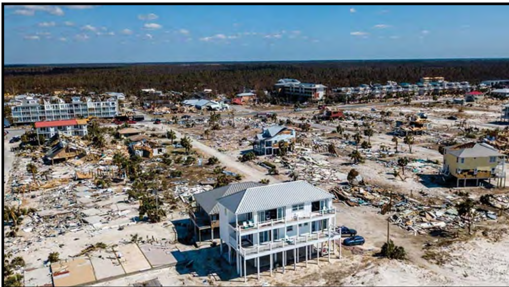
ICF home surviving a 250mph hurricane on Mexico Beach Florida
